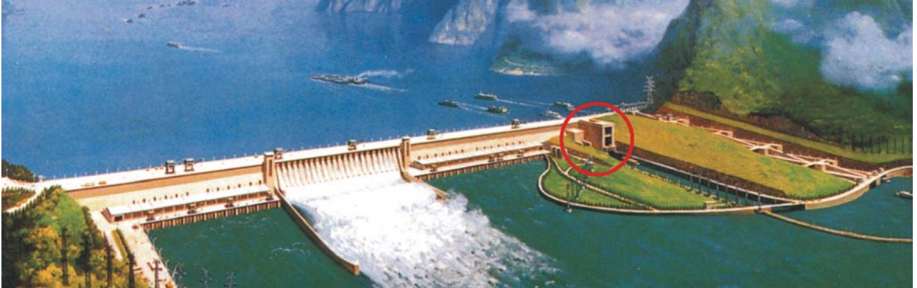
Visualisation of the overall project with marking of the planned ship lift
