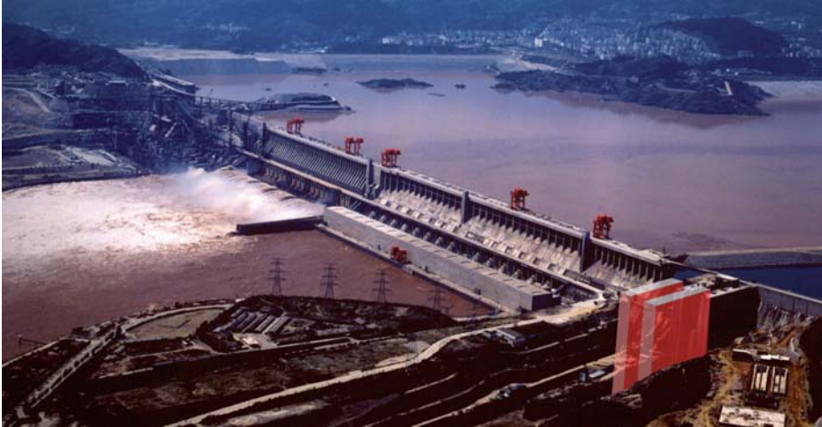
Overview of the overall construction with marking of the contours of the ship lift in 2004
