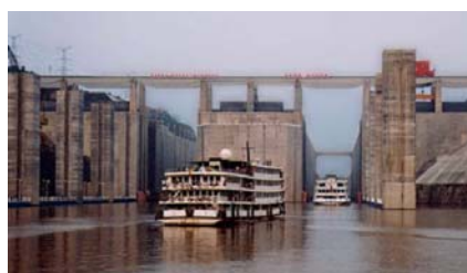
Upper lock access with view into the lock chamber of the double lock
