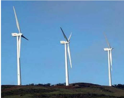
These wind turbines on the island of San Cristobal in the Galapagos are part of a certified Clean Development Mechanism wind-diesel hybrid system to reduce use of diesel fuel. (Photo courtesy Galapagos Wind)
