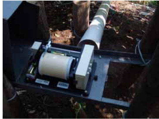
Figure 8 Extensometer installed in Shuping landslide The deformation is recorded on the rolled paper (left) and also saved in a memory (right box)
