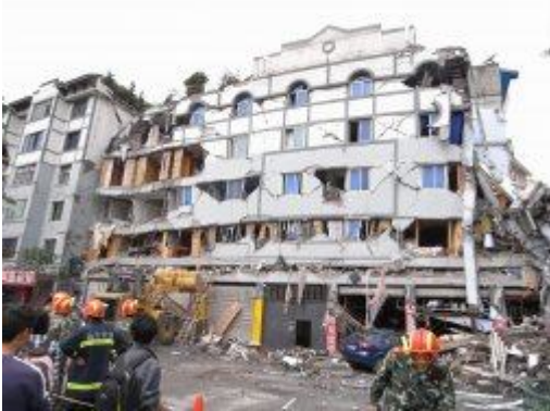
Sichuan earthquake damages building, 14 May 2008 ( Miniviki )
